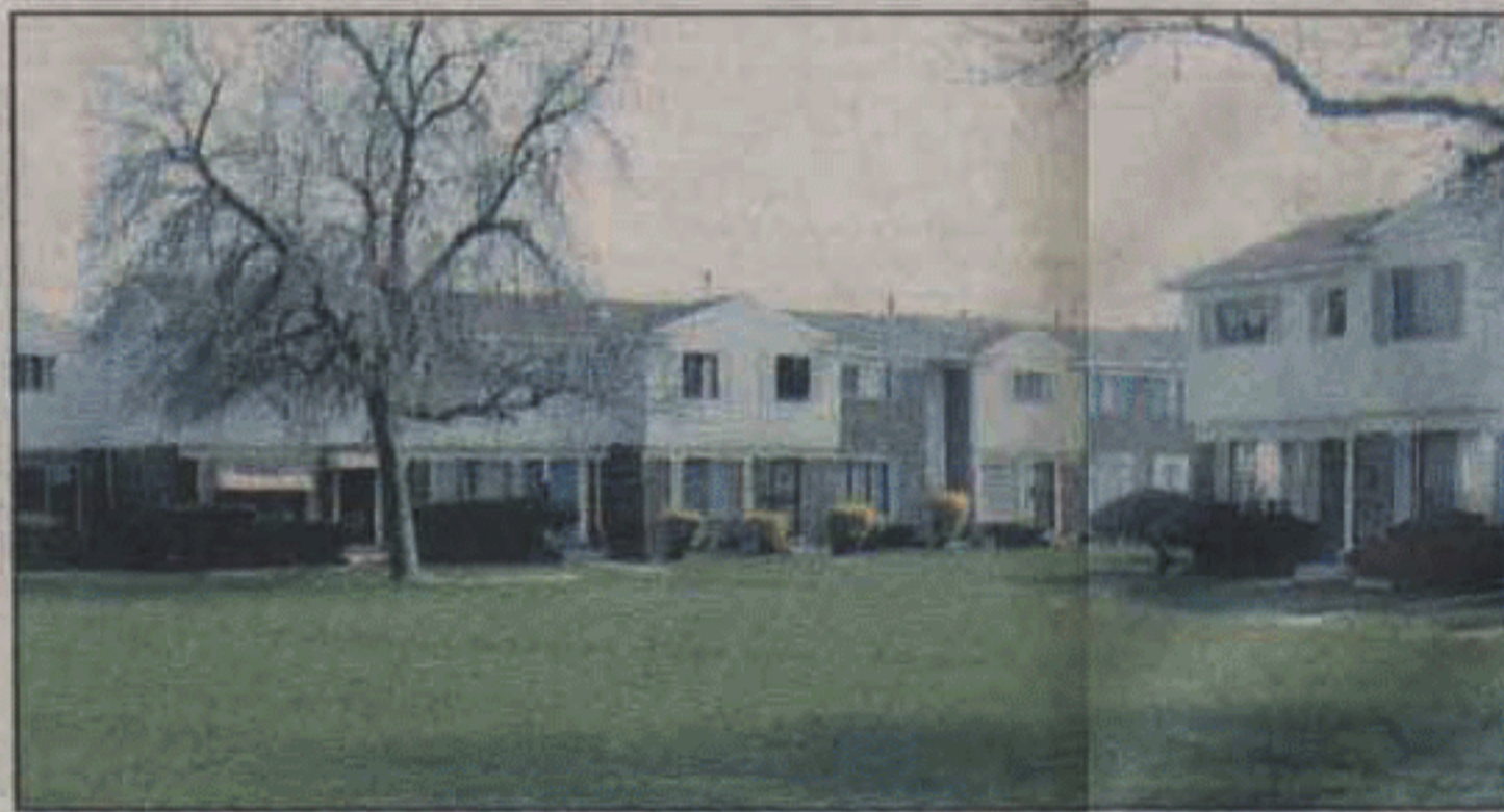
The London Towne Houses Cooperative at 830 E. 100th St.
