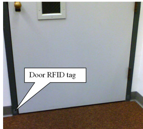
Figure 2. RFID tag describing a door
